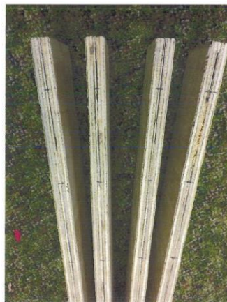
Figure 3: Drill 24 holes (6 per rail) in Main Rails
